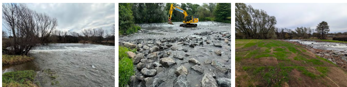
Figure 16. Stages of the weir mitigation on the River Leven.
